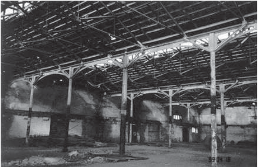
Figure 7.2 Interior Structure of Stack A Prior to Redevelopment
